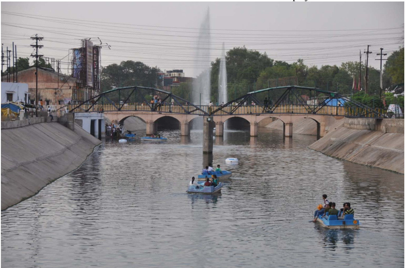
Photo 12. June 2011: Recreational area of the Swarn Rekha River after Sub-project intervention
