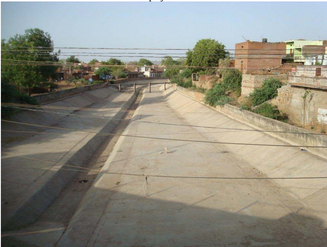
Photo 2. April 2010: Lined river bed after Sub-project intervention
