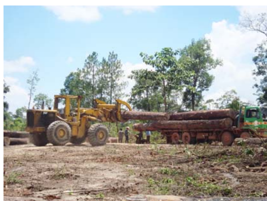
Sub contractor moving VFA logs, near Ban Done
