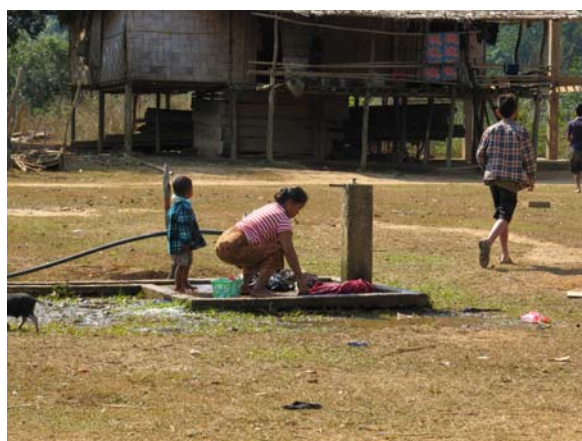
Water point, Ban Sam, NPA, Southern Zone, installed by WMPA.
