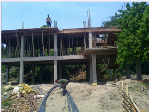
Construction begins on the new OCR building.
